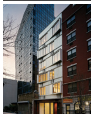
17 Switch Building nARCHITECTS 109 Norfolk Street
